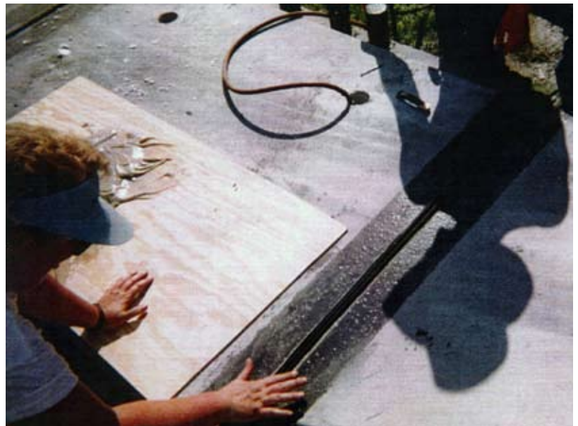
WaboCrete II is installed on the test track
